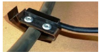
Sensing probe connected to generator ground cable
